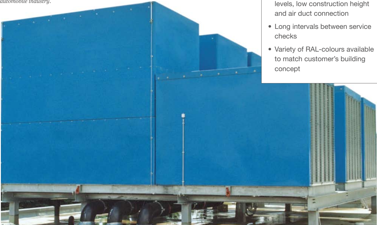
Figure 5: Forced-draught cooling tower Type EWK-D cools a transmission test bench in the automobile industry.
