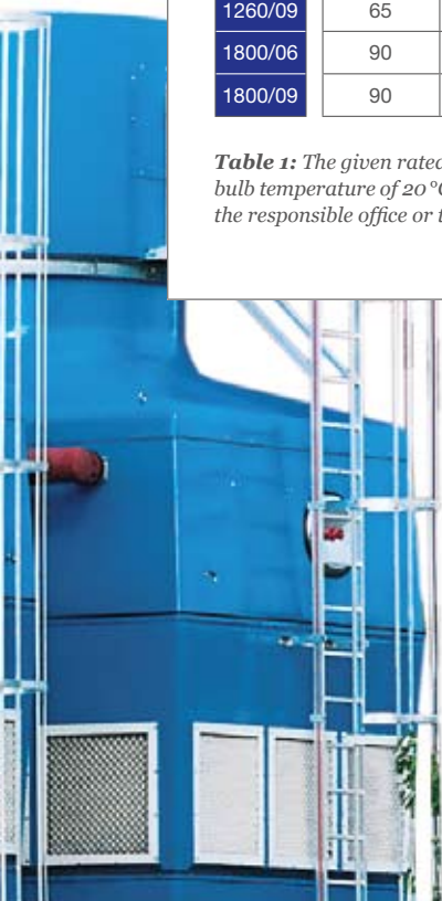
Figure 2: Two intake, ventilated cooling towers Type EWK 1260 guarantee the process cooling for the automobile supplier.
