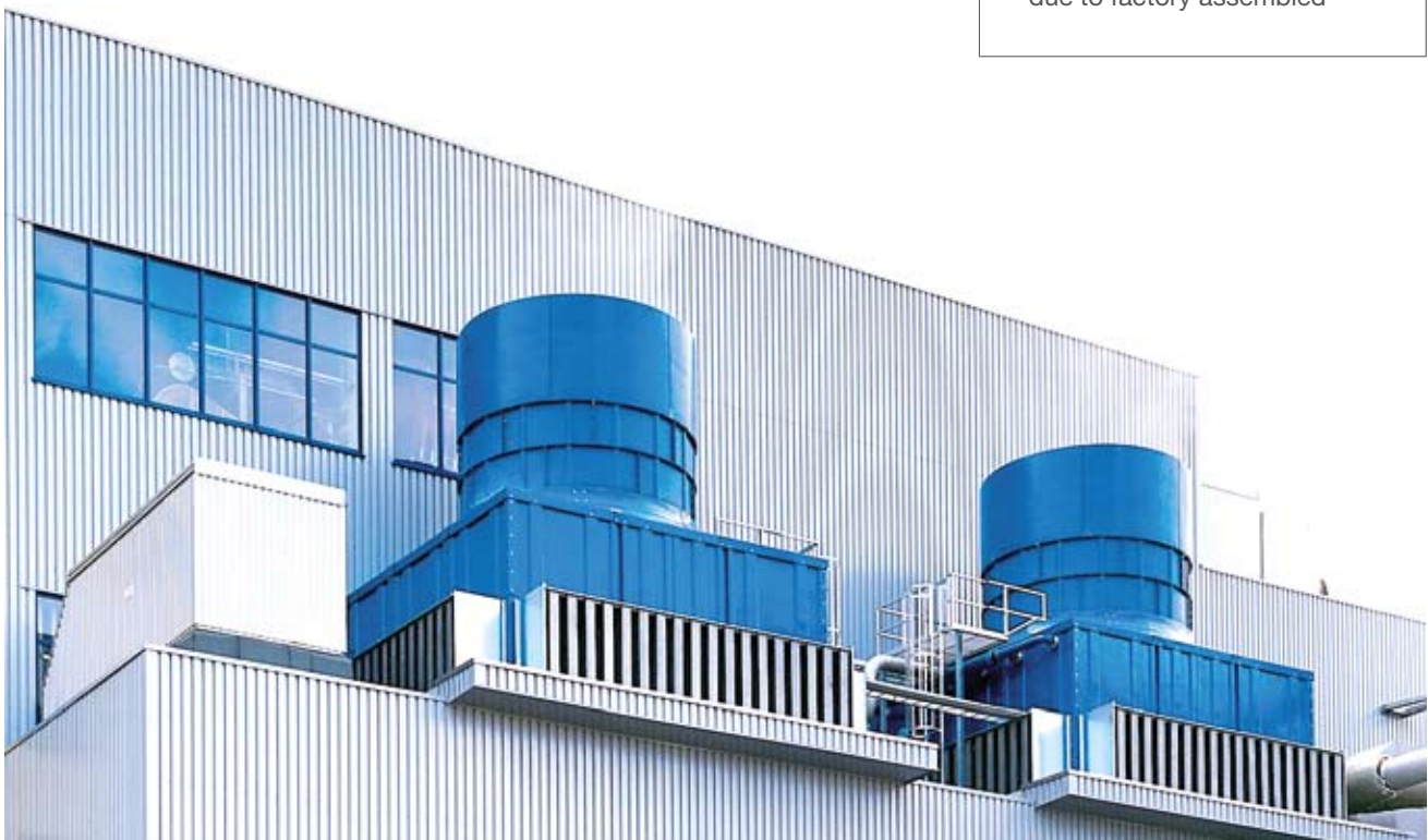
Figure 3: Two MODUPOL® cooling towers to cool processing water with a special ventilator, plus air supply and outlet noise-reduction.
