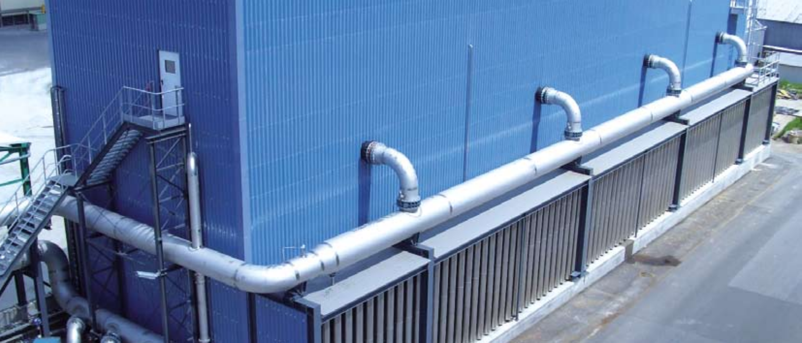
Figure 6: Cell cooling tower system Type EWZ 119.
