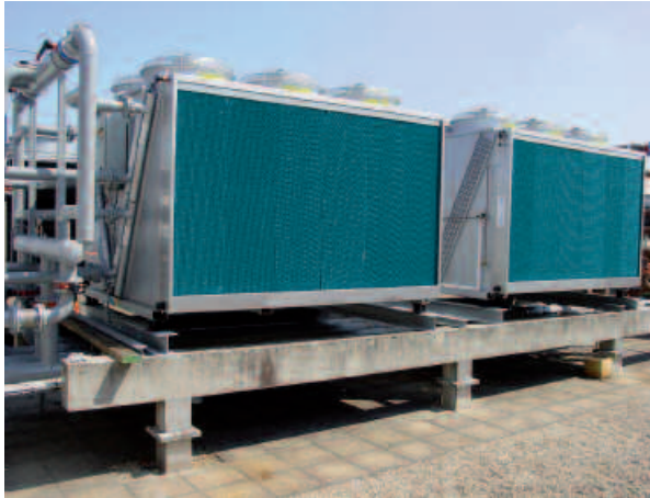
(Right) Close-up of an EPCC. Here it can be seen that a metal frame holds the pre-cooler high performance media. (Left) Each installation has its own special requirements as can be seen from the placement of pre-coolers on a refrigeration system on a building complex in La Habahera.
