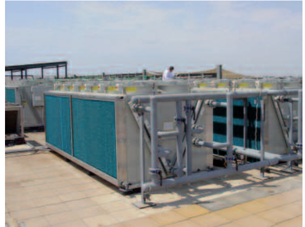
(Right) Close-up of an EPCC. Here it can be seen that a metal frame holds the pre-cooler high performance media. (Left) Each installation has its own special requirements as can be seen from the placement of pre-coolers on a refrigeration system on a building complex in La Habahera.
