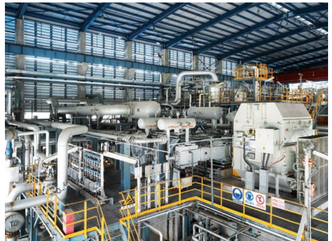
LDPE compressor train: Process Gas Compressor and Hyper Compressor at 3'100 bara (45'000 psia) by Burckhardt Compression – the global technology leader in the reciprocating compressor world
